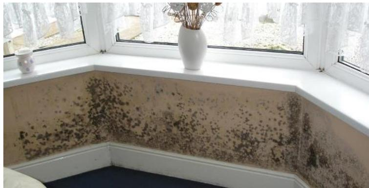
This is damp caused by a leak somewhere. This needs reporting to the Agent / Landlord so repairs can be carried out. Let us know what you think is causing this leak so we can send out the correct workers.
